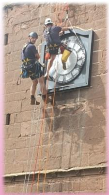
The reinstalled fully electric clock is now set within a metal surround rather than wood as it once was. The whole task, including pointing the area behind, was completed without sight of ladder nor scaffolding!
